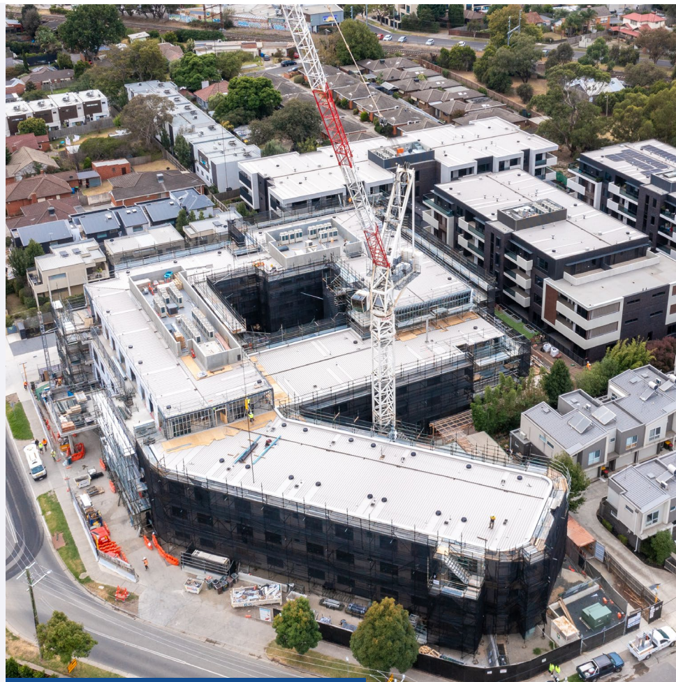
Bert Newton main building under construction, 7 March 2024
